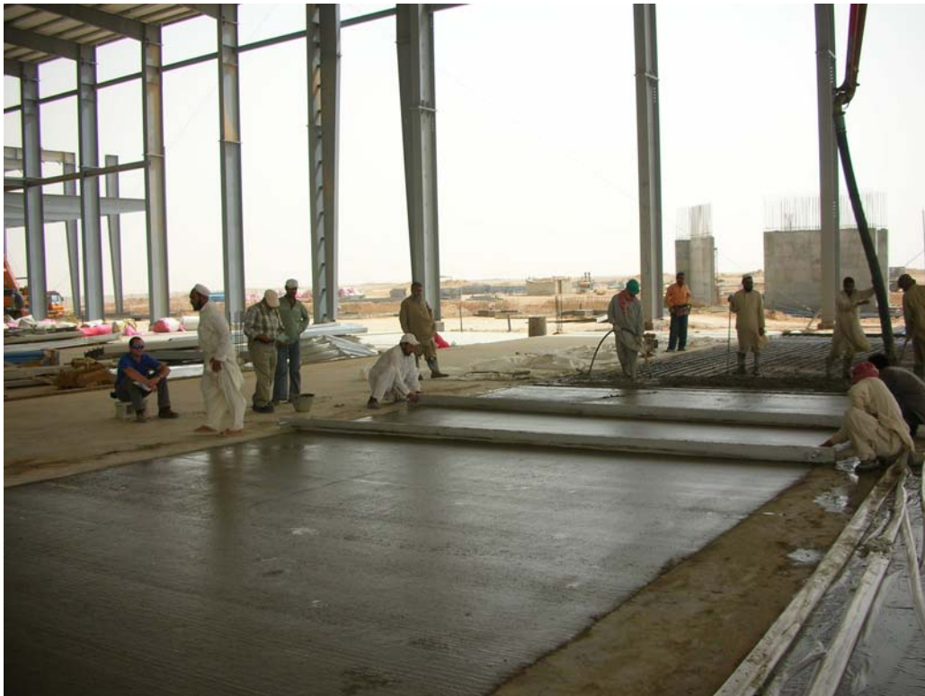
Long Strip construction- Typically 4 – 5 m wide
