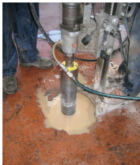
FACE-CONSULTANTS WORKERS TESTING FLOOR STRENGTH AND STABILITY.
