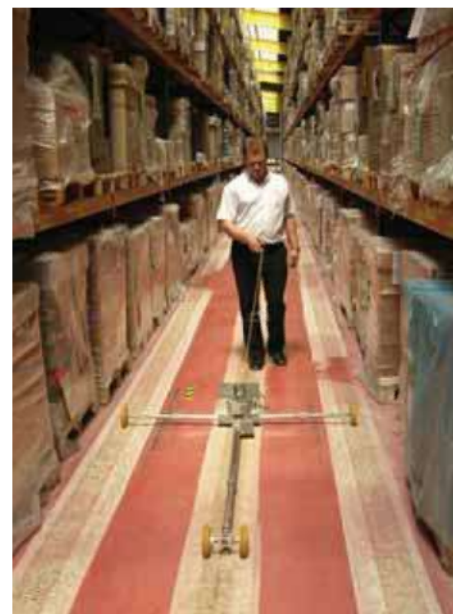
A Concrete Grinding operative using a profileograph to measure floor flatness.
