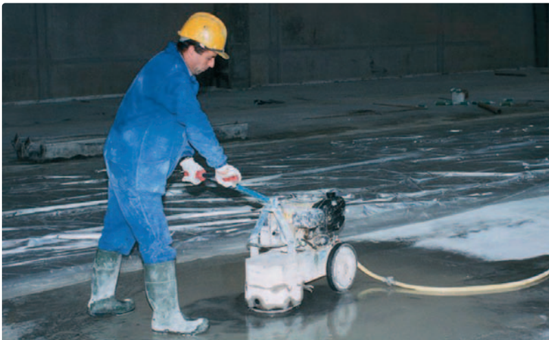
Figure 1: Walk-behind manual grinding.
