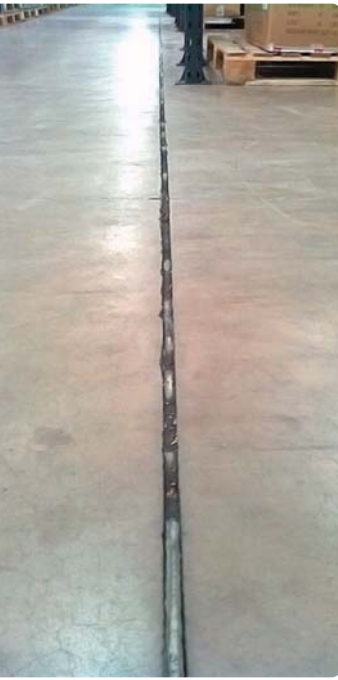
Figure 1: Sawn joint in a free movement area.
