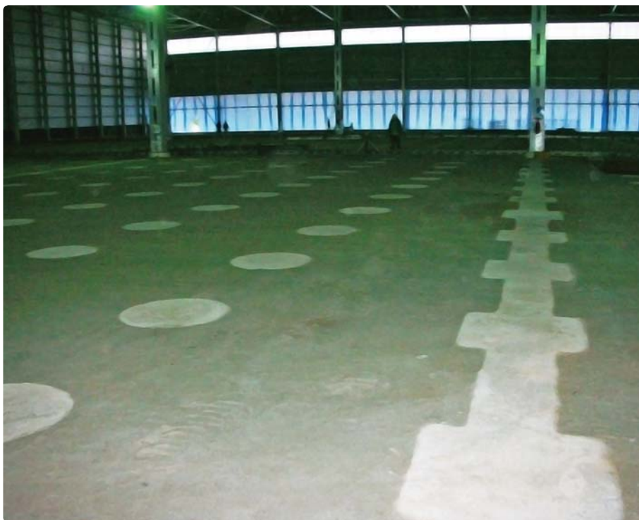
Figure 7: Pile heads and sub-base.
