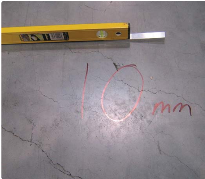
Figure 3: Deflections at mid span.
