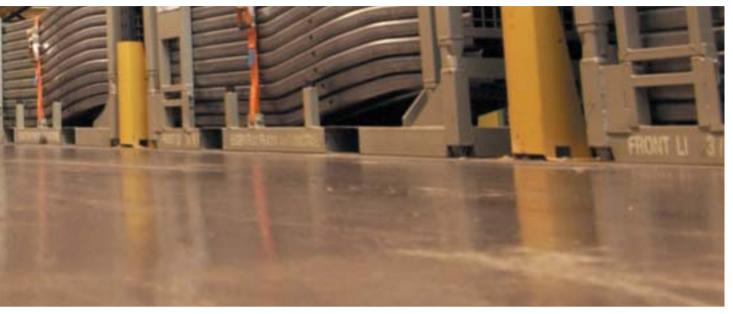
in the UK and Europe are of three-wheel configuration and feature centrally positioned single or close-coupled rear wheels. At present the effect of these wheels on the performance of a truck is not considered when a warehouse floor's flatness in relation to the operation of VNA machines is being assessed.
