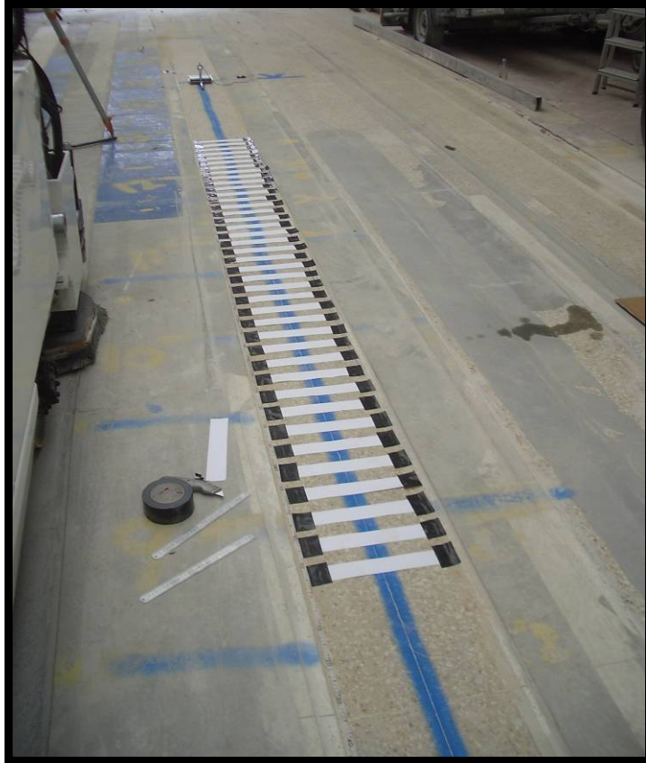
Fig. 5 – The strips were laid out between 2 and 6 metres (4 metre length)
